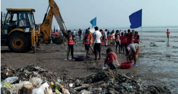
The mound of trash in the foreground will be transported by tractors to the waste segregation center
